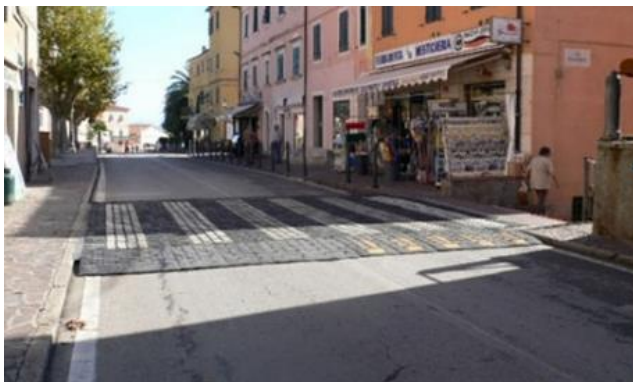
Figure 3: Rubber pedestrian crossing in the provincial road
